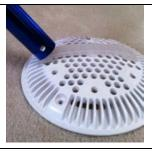
(7) Use the utility pole as pictured above to push on the end of the clip and securely "seat" the hook into the holes.
